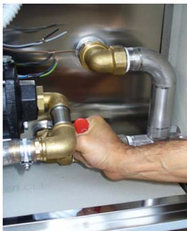
***Turn the control lever in horizontal position as showed in the picture***
