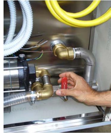
**After cleaning the water tank close the auxiliary tap and turn the control lever in the original position as showed in the picture**
